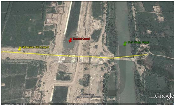
Figure1, Damages of Kachhi Canal due to Mithawan hill torrent flow.
